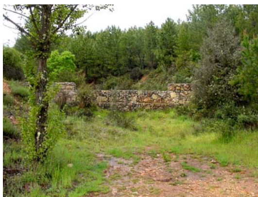
Fig. 3. Stabilisation dike made of gabions
