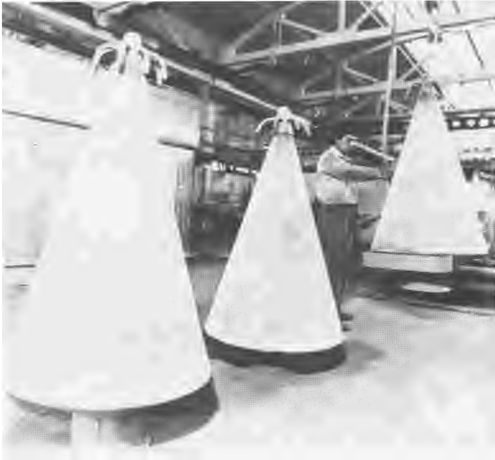
Plate 6. Fish-protection intake with a flow-former
