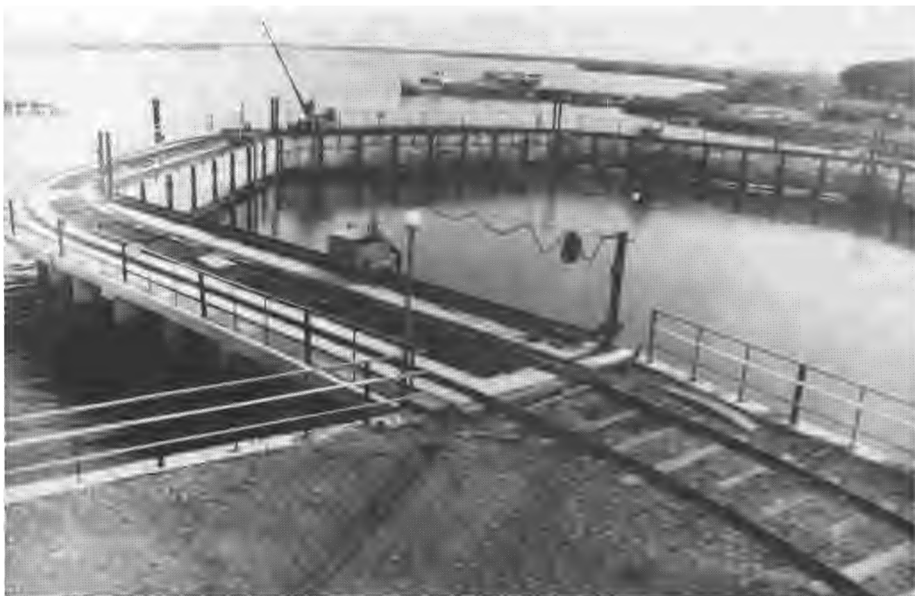
Plate 3. Fish protection screens with movable screen elements.
