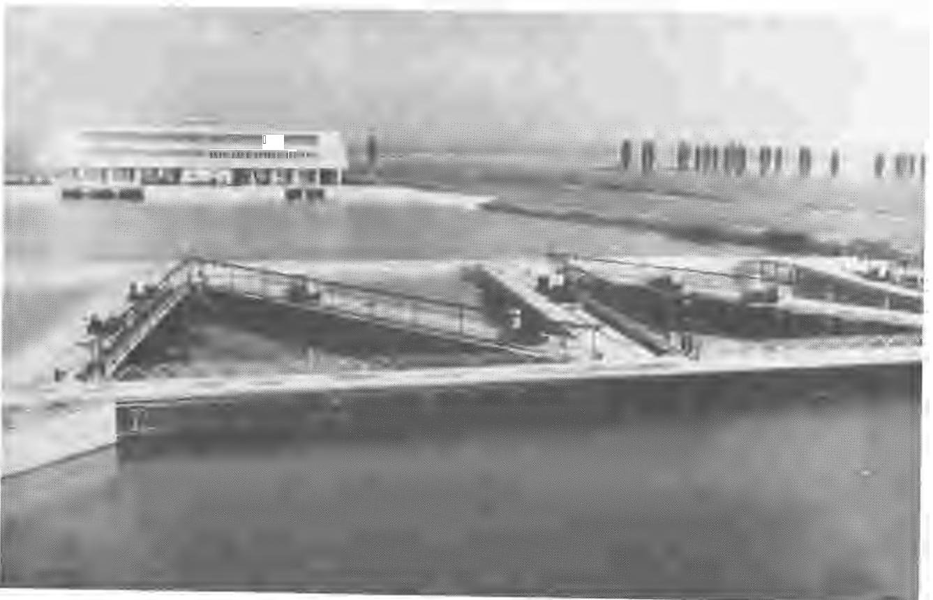
Plate 9. Conical fish-barriers with fish-diverting devices.
