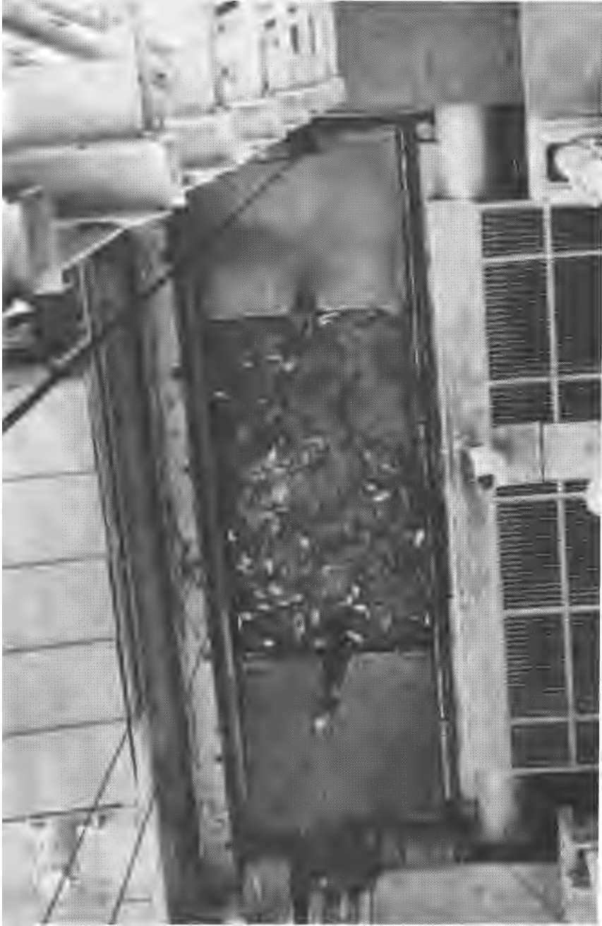
Plate 1. Fish retention grid of the Krasnodarskiy fish-lift on the Kuban' River.
