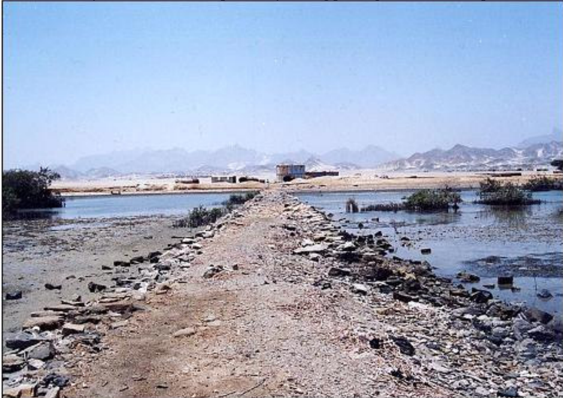
Photo 12 - Jetty built at El Hamirah potentially causing ponding of waters and impacts the mangroves.
