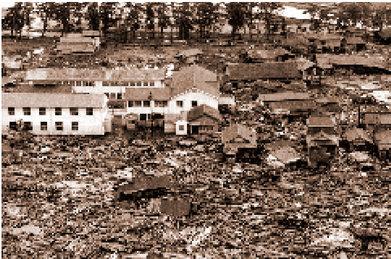
A narrow shelterbelt of pine trees near Shizugawa (Miyagi Prefecture), Japan appears to have protected the houses within its shadow during the 1960 Chilean tsunami. Waves came from the Pacific (top of photo) and river mouth (left side of photo). Destruction in foreground also includes debris left by river inundation.
