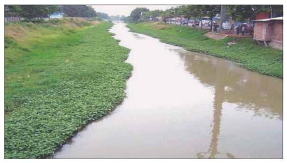
Figure 5. Weeds in unlined canal
