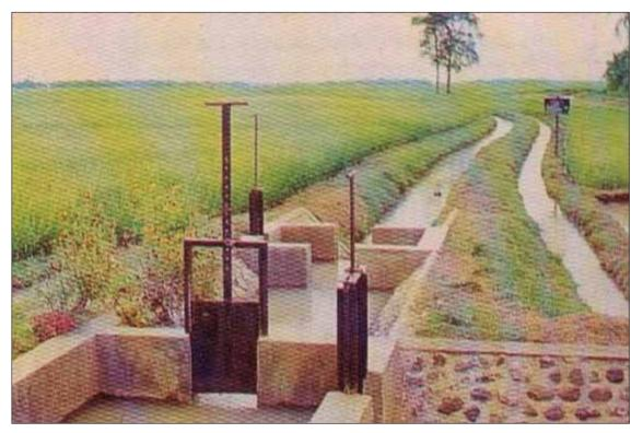
Figure 3. Distribution structure and tertiary canal
