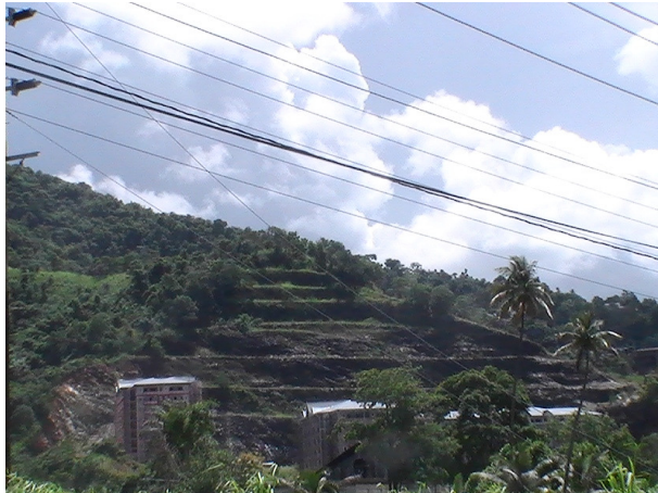
Photograph 6. State terracing of slope to protect construction
