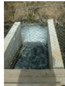
Water outlet, screened for avoiding penetration of otters
