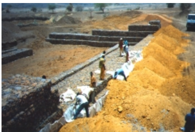
PLATE 7.18 Using earthfill and geomembrane to waterproof the weir
