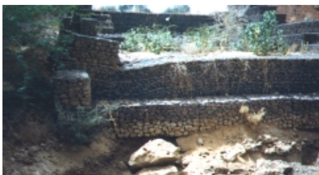
PLATE 9.2 Scour damages to gabion structure
