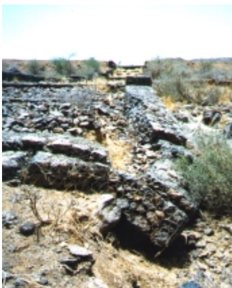
PLATE 9.1 Settlement damage to gabion structure
