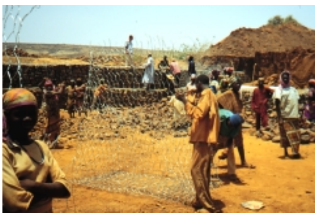
PLATE 7.13 Opening the gabion net
