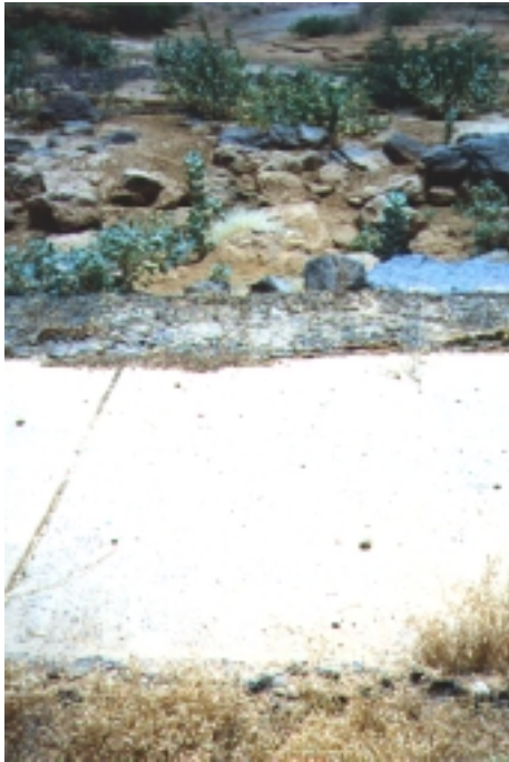
PLATE 7.20 Stilling basin lined with reinforced concrete
