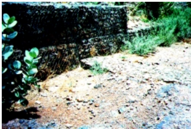
PLATE 5.1 Linear protection of gabions on channel floor
