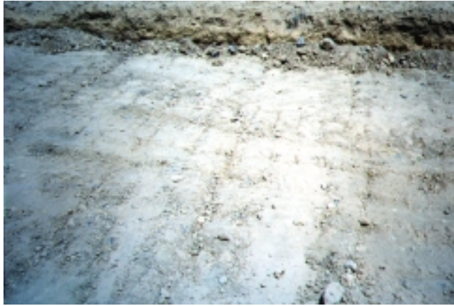
PLATE 7.6 Scarifying the top of a layer
