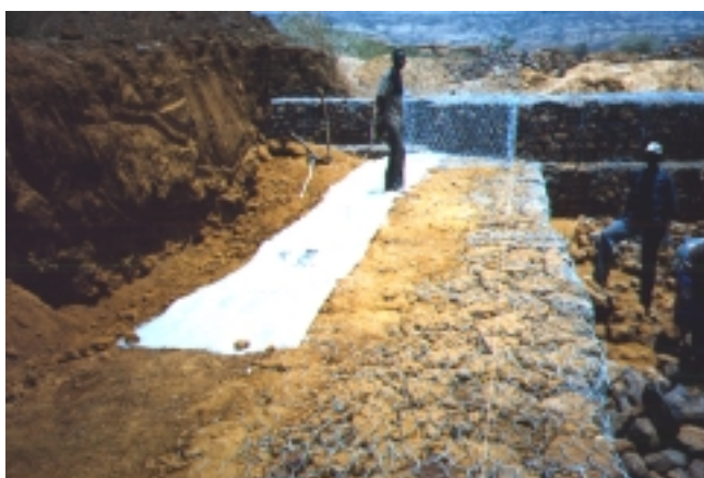
PLATE 7.12 Placement of geotextile
