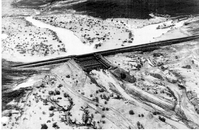
PLATE 1.4 A central spillway using gabions
