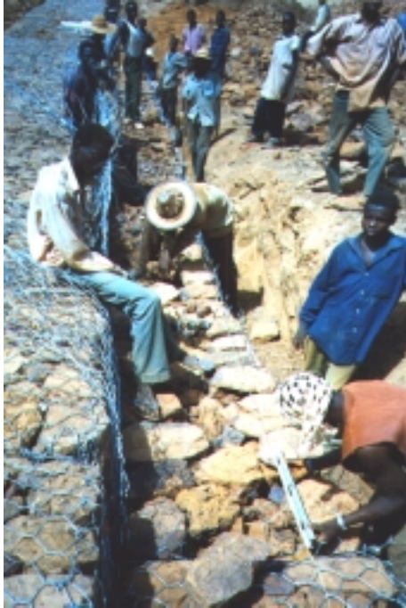
PLATE 7.15 Verifying the top level before closing
