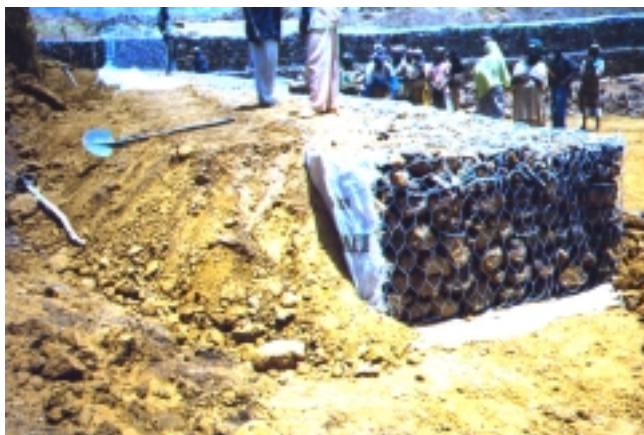
PLATE 7.17 Fill compaction next to the gabion
