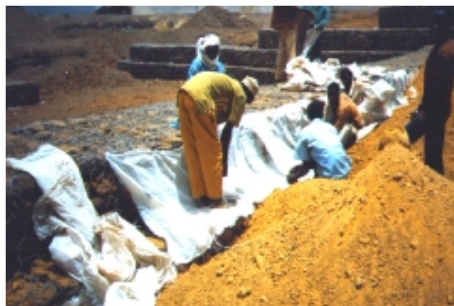
PLATE 7.19 Placing the geotextile
