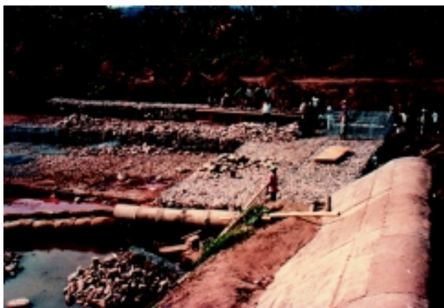
PLATE A1.2 Gabion apron under construction with the dewatering arrangement
