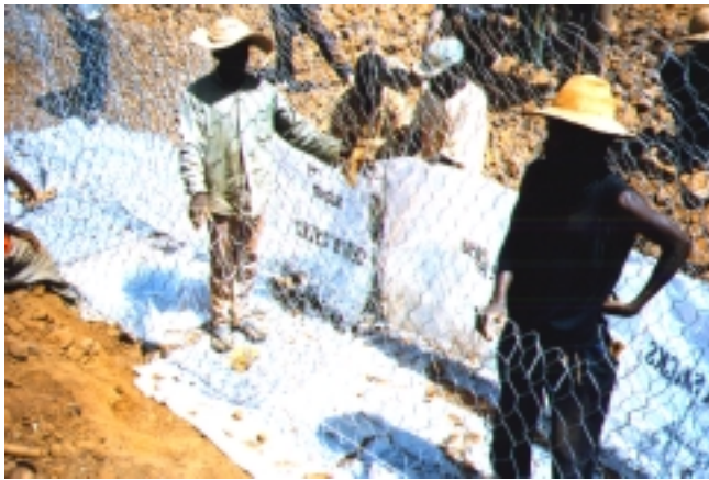
PLATE 7.22 Semi-permeable cut-off screens
