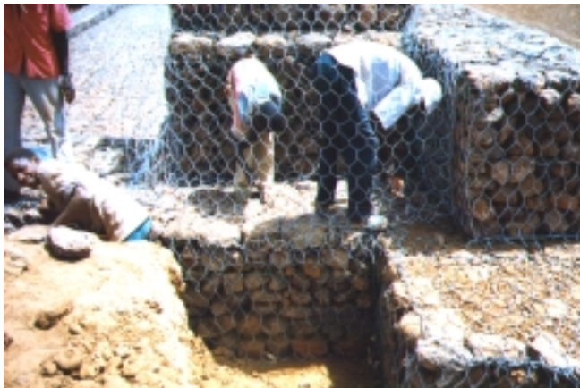
PLATE 7.16 Superimposing gabion layers
