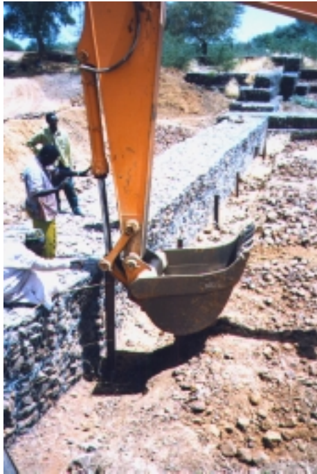
PLATE 7.21 Lining and anchoring a counter weir
