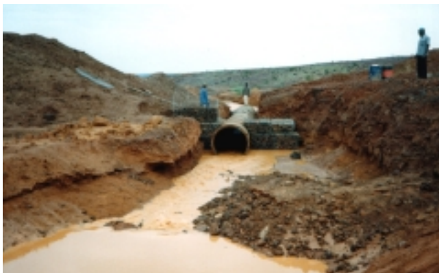
PLATE 7.1 Runoff passing through pipeline inserted in the earthfill during embankment construction
