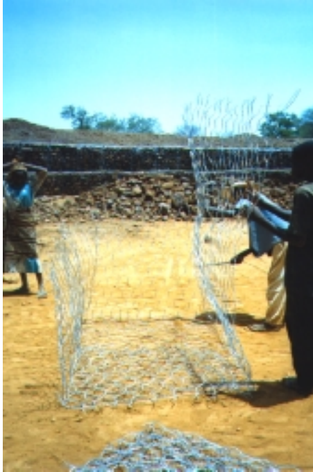
PLATE 7.14 Assembling the gabion baskets
