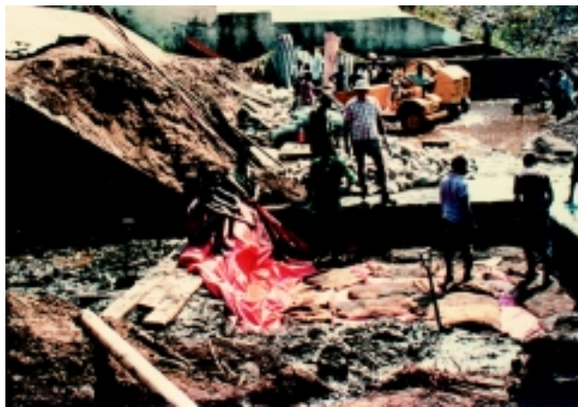
PLATE A1.1 Laying plastic sheet on top of sand filled bags
