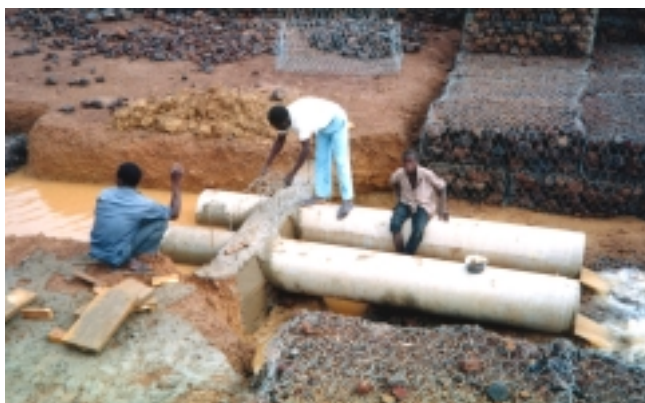
PLATE 7.8 Preparation of cut-off collars
