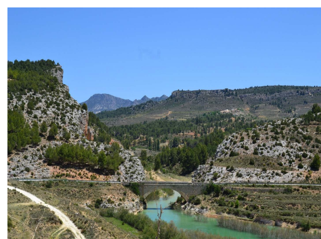
Fig. 3: The alluvial wedge behind the check-dam creates a sediment sink and thus an opportunity to sequester carbon. Protection of soils through proper management is important to decrease connectivity
