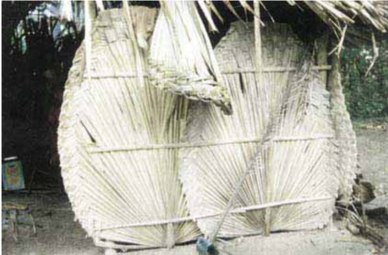
Figure 4-7 House wall panels made from buri leaves (Corypha utan). Mindanao, Philippines. Photograph by Dennis Johnson.
