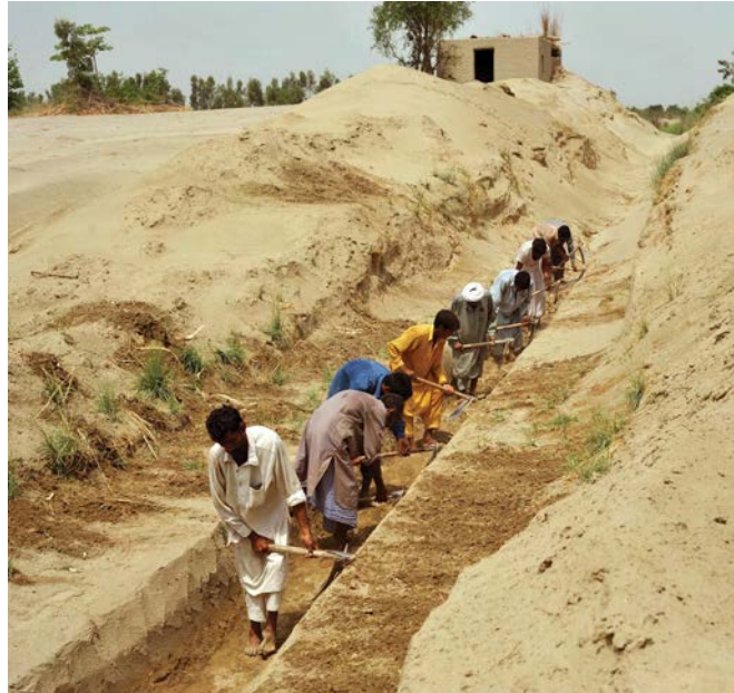
Farmers in Pakistan digging a water canal in the sand
