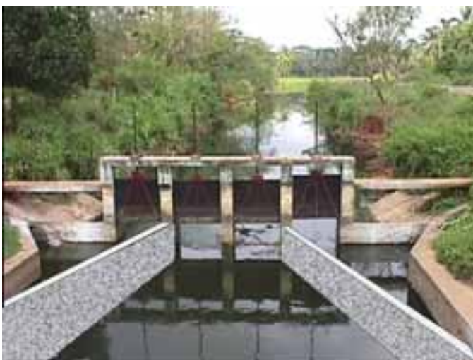
Plate 31 Building side weirs on gated regulators.
