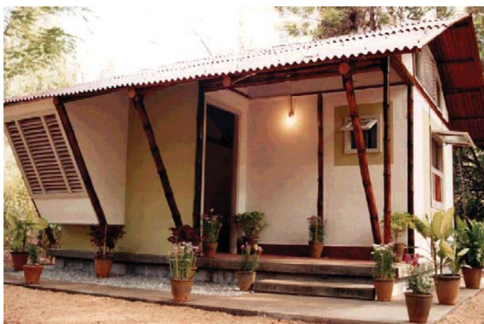
10. Prefabricated bamboo house, India (INBAR)
