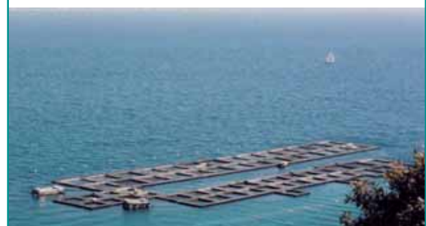
FIGURE 16 Cannes Aquaculture (France) using floating cages built with Jetfloat components
