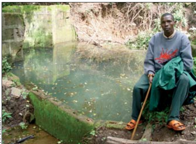
An impoundment constructed about 30 years ago collects Mount Kulal spring water which is then piped to holding tanks that serve local communities
