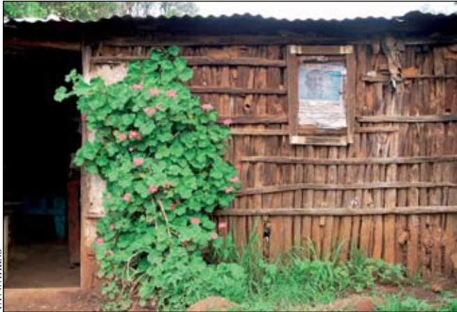
Construction of houses from wood is the most common use of forest products in the villages of Mount Kulal
