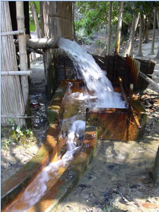
Figure 3. Irrigation water discharging from pump into concrete channel, showing orange Fe oxide deposition as water oxidizes
