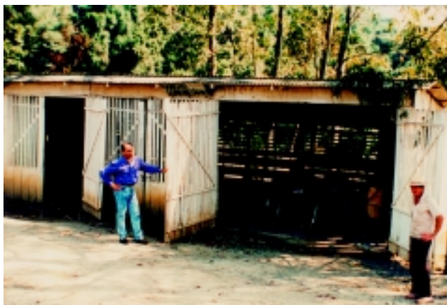
PLATE 49 Machinery barn for community use - an example of self-management of the development process
