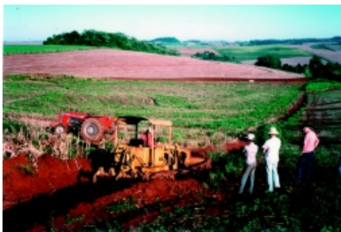
PLATE 45 Commencing the process of gully elimination
