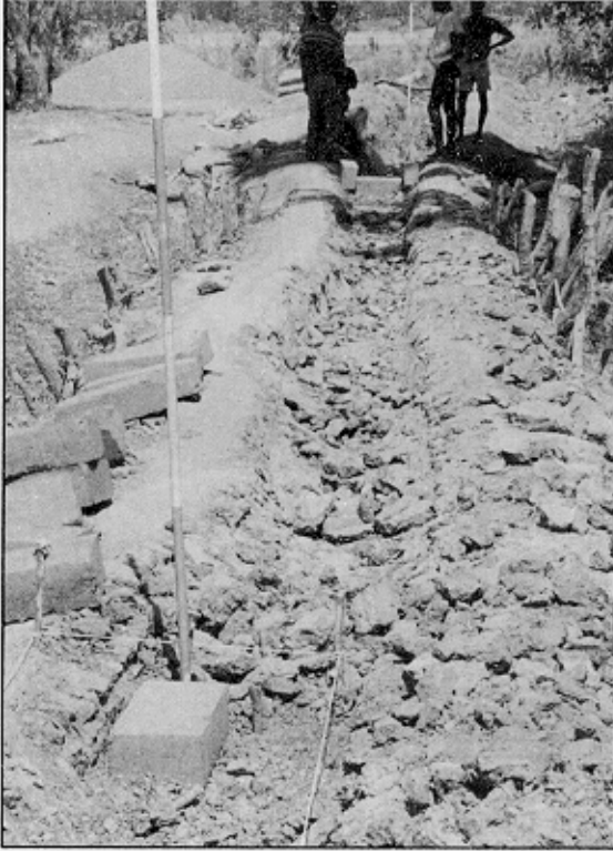
FIGURE 44-A Destroying the old canal bed
