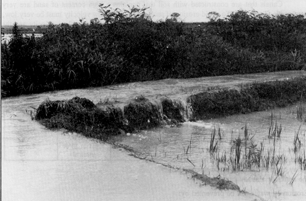
FIGURE 26 Eroded canal
