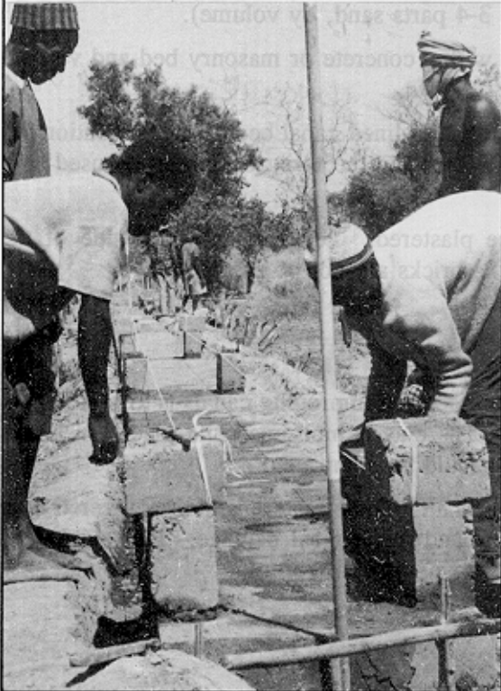
FIGURE 44-C Making the walls
