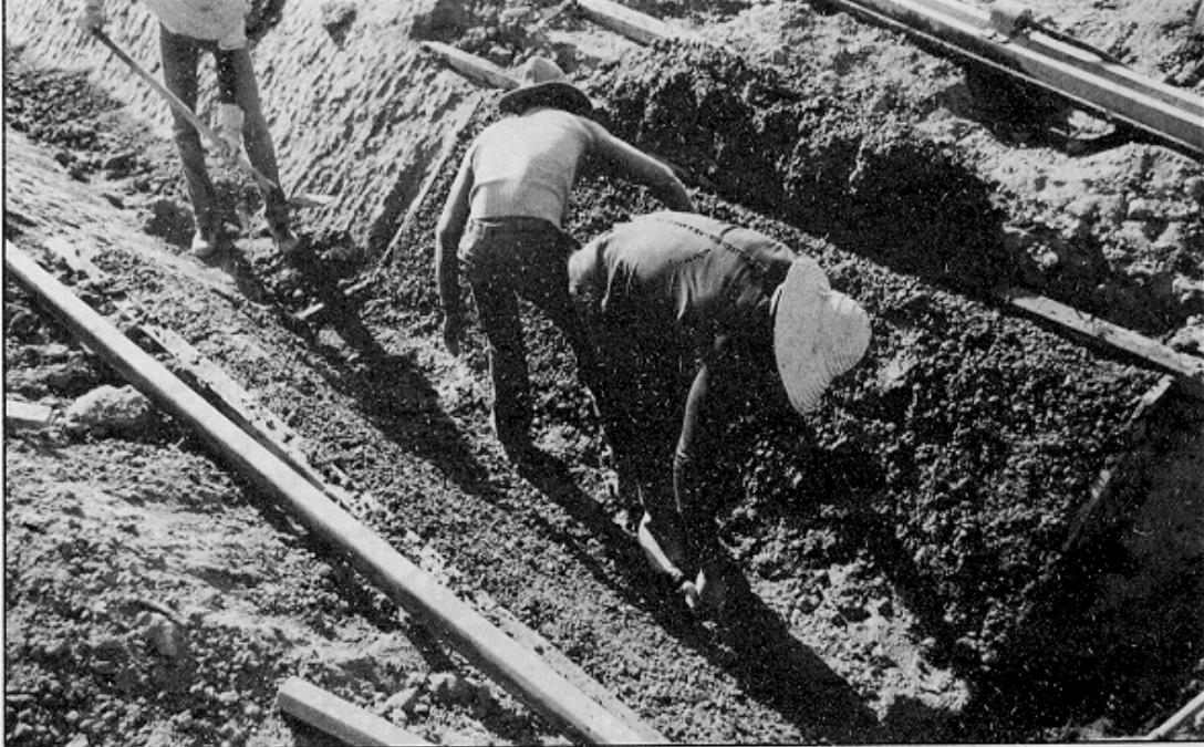
FIGURE 42-B Pouring the concrete
