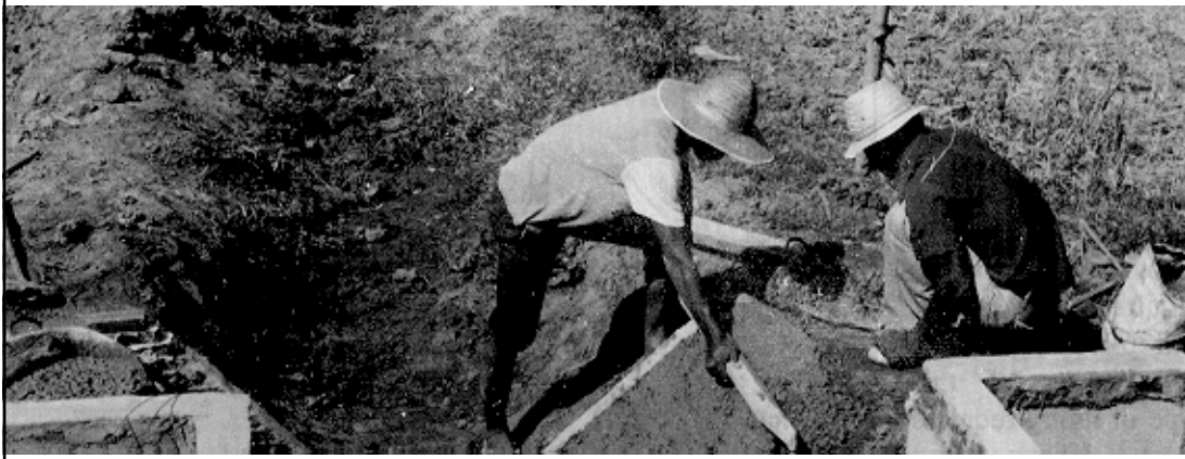
FIGURE 41 Hand plastered canal lining
