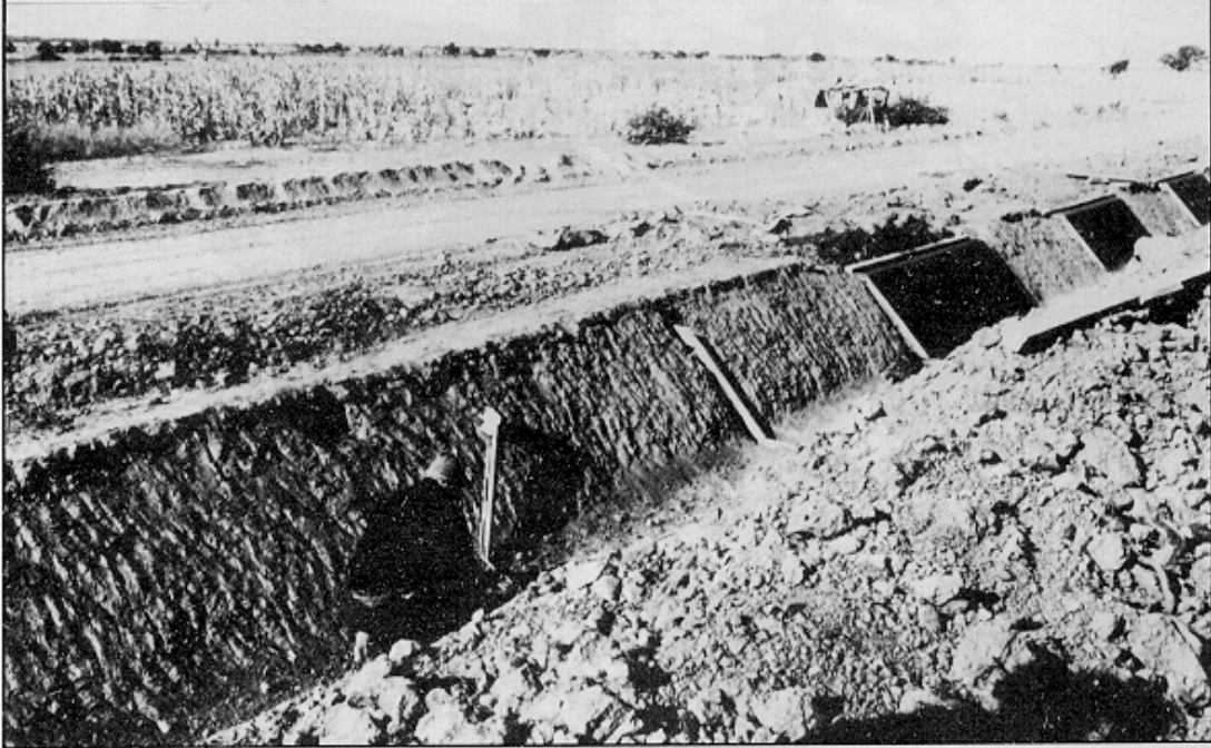
FIGURE 42-A Installation of guide forms
