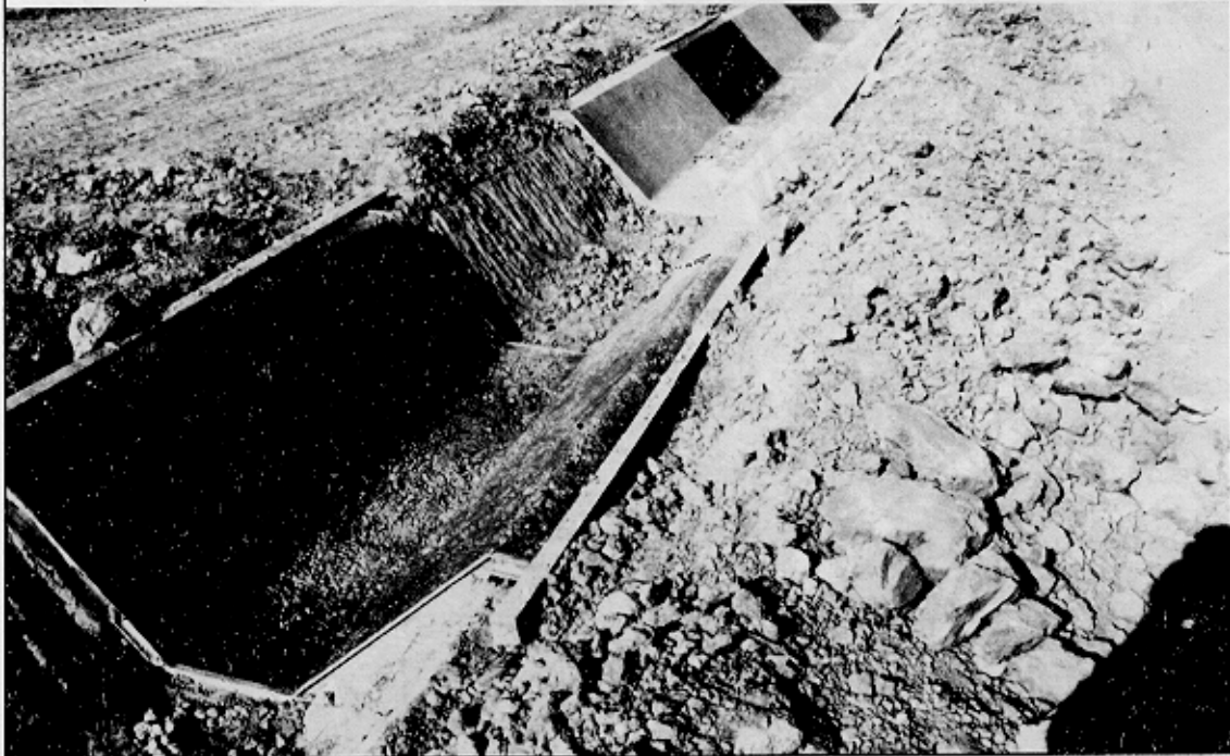
FIGURE 42-D Alternately lined canal sections
