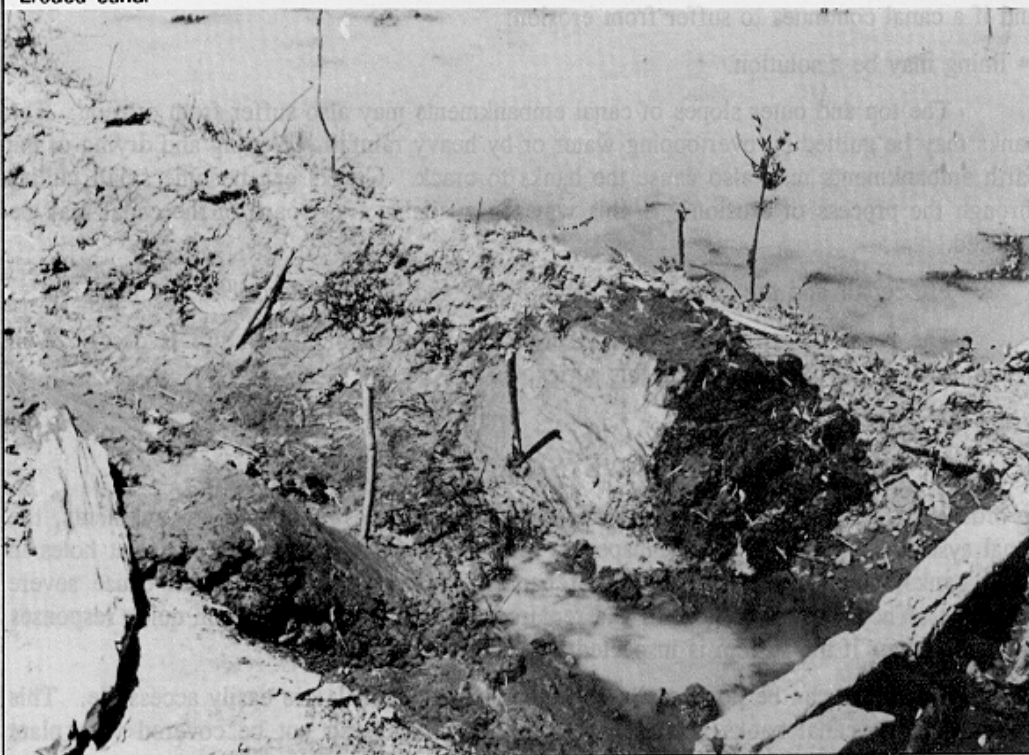
FIGURE 26 Eroded canal
