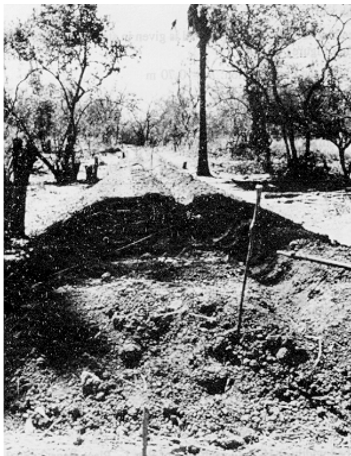
FIGURE A2.8 Embankment under construction
