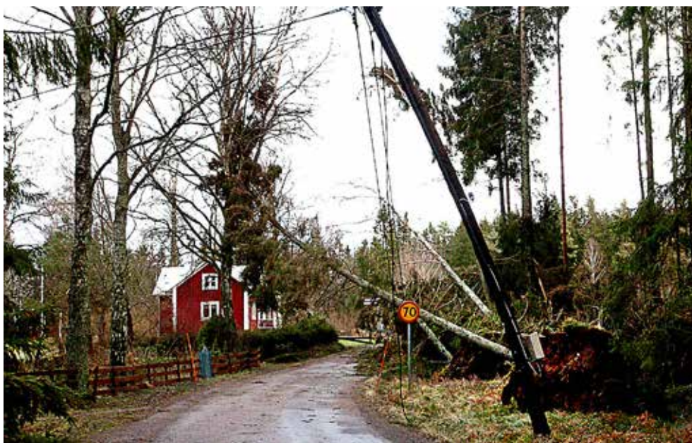
PHOTO 21 Telecommunication and electricity breaks were rampant after the Gudrun tempest in January 2005.
