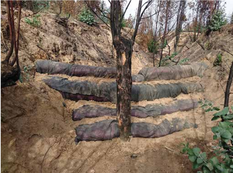
Erosion control structures built by Arauco near Santa Olga to safeguard water quality
