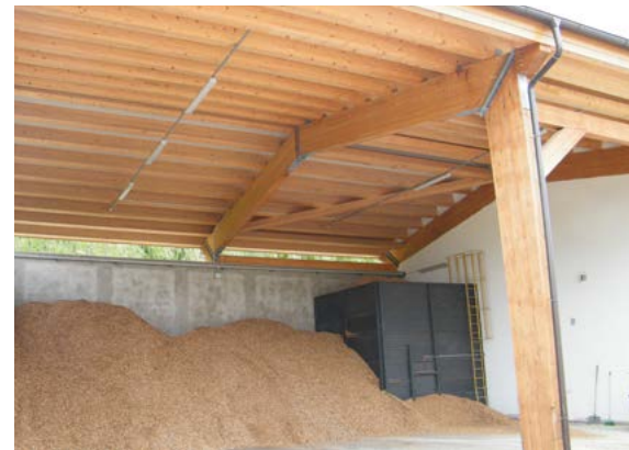
Figure 33 and 34: Covered chip storage and open ground material storage
