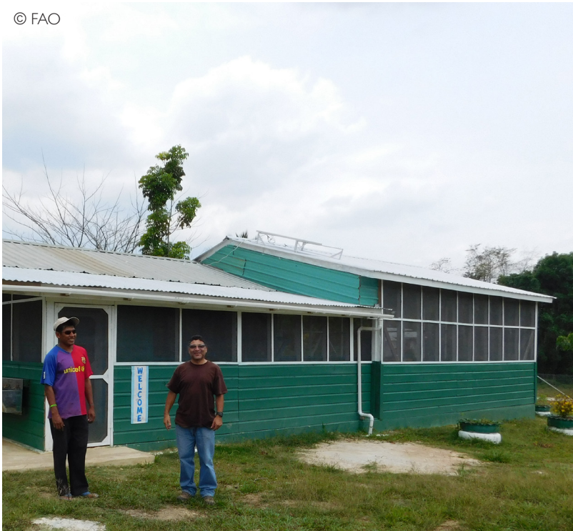
© FAO New kitchen, storage and lunchroom area, November, 2016.
