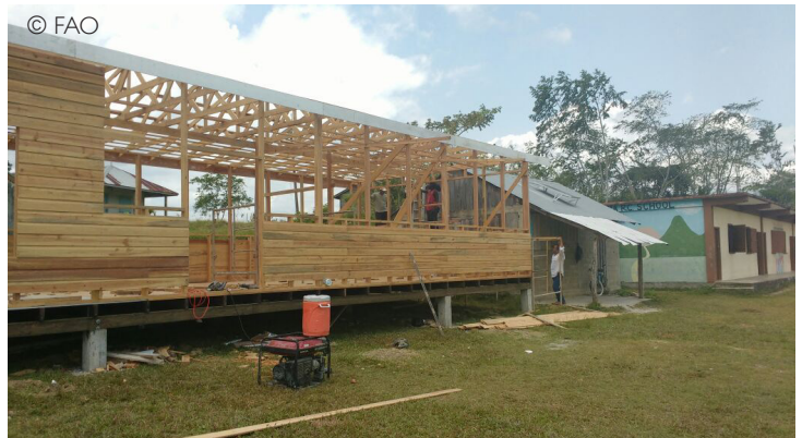
Kitchen, storage and lunchroom. Construction in process, July 2017.
