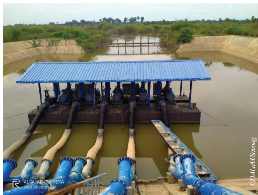
Head irrigation with electric engine at Hardxayfong.
