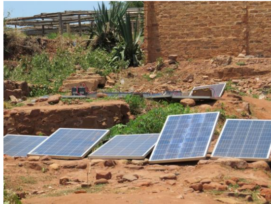
FIGURE 52. SOLAR ENERGY USED TO CHARGE THE BATTERIES THAT POWER THE LIGHTS USED DURING NIGHT FISHING
