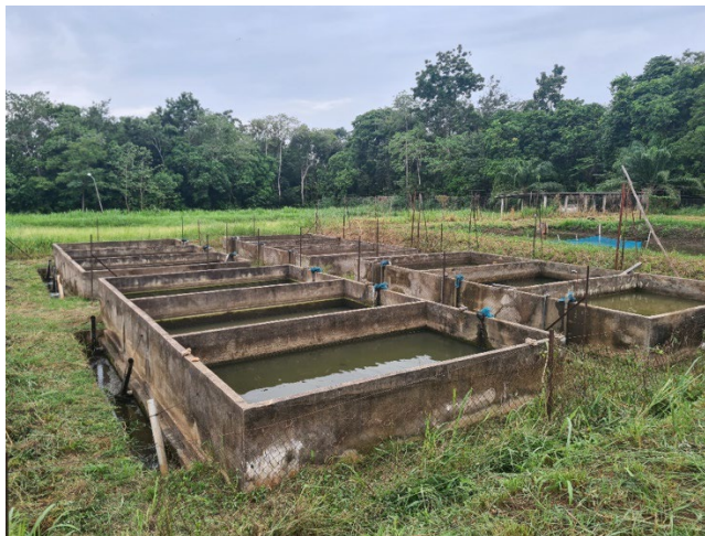
Figure 13 - Installation du CNRA
