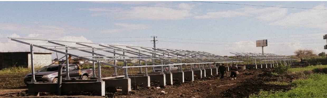
Al-Afir project – double post mounting structure FAO, 2017, El- Behiera Governorate, Egypt
