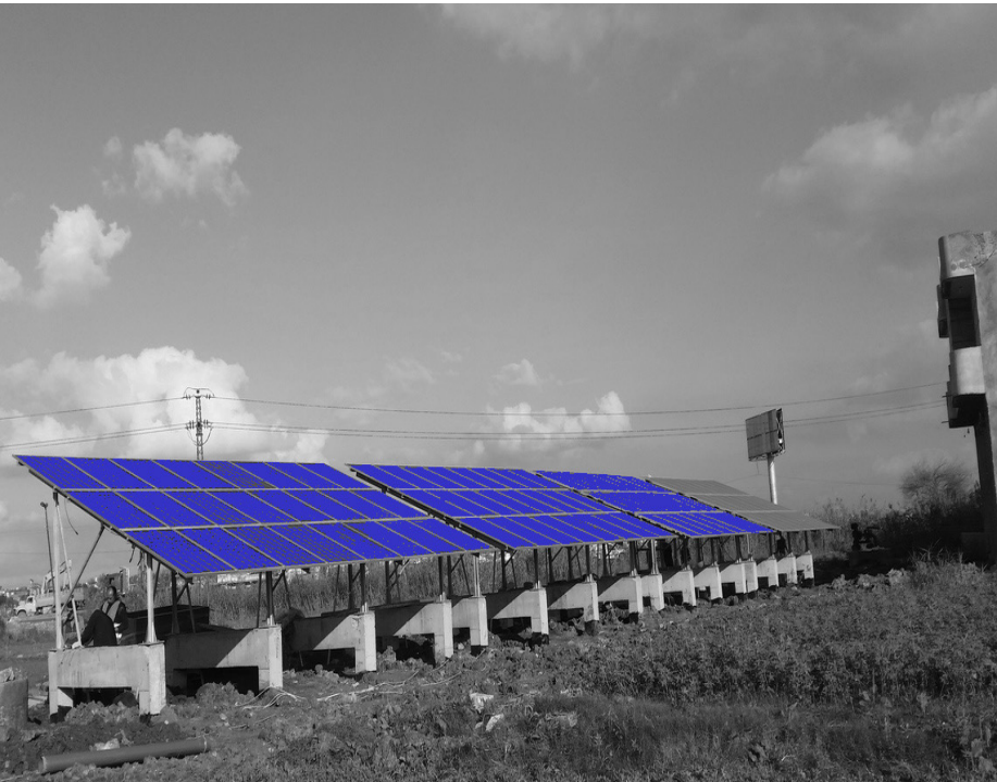
Al-Afir project – Solar powered irrigation system in the Nile Delta, Source: FAO, 2017, El- Behiera Governorate, Egypt
