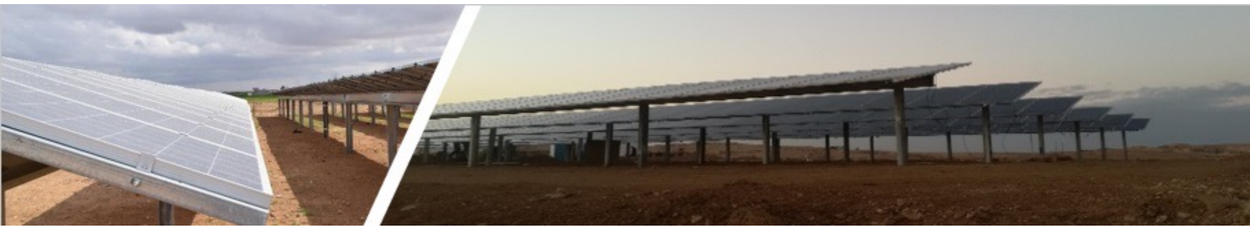
Single post mounting structure _Al Ghadeer Al Abyad project Source: FAO, 2018, Al-Mafraq Governorate, Jordan
