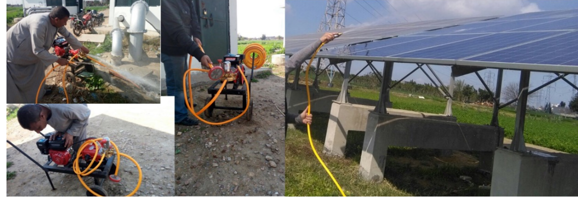
training session on the cleaning of PV modules for the beneficiaries of FAO's Al-Afir project, El- Behiera Governorate,
