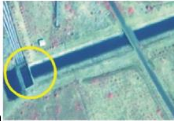
Main canal offtake
