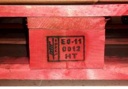
Mark, applied with a fire-brand stamp, is similar to example 2 of Annex 2 of ISPM 15 but producer/treatment-provider code is split over first and second line
