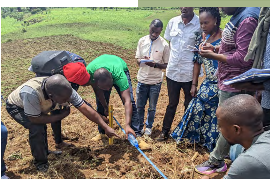
Implementation of erosion control as a restoration option, pictured here in Mulungu, determining the slope of the land with local materials (used water bottle). © FAO/Floribert Mbolela
