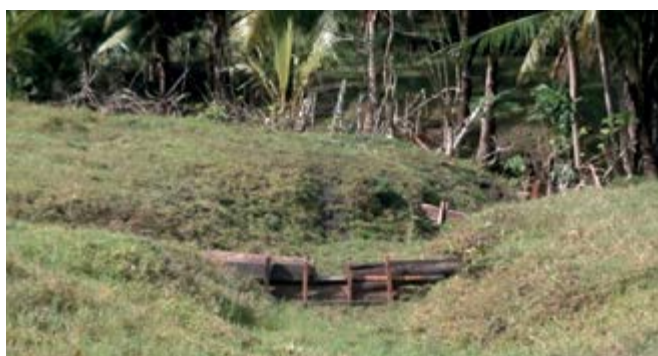
Livestock farm in the province of Los Santos. Gullies plugged with wooden barriers to retain sediments.
