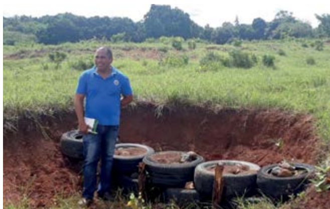
Livestock farm in the province of Herrera. Earth barriers made from old tires to heal a gully.
