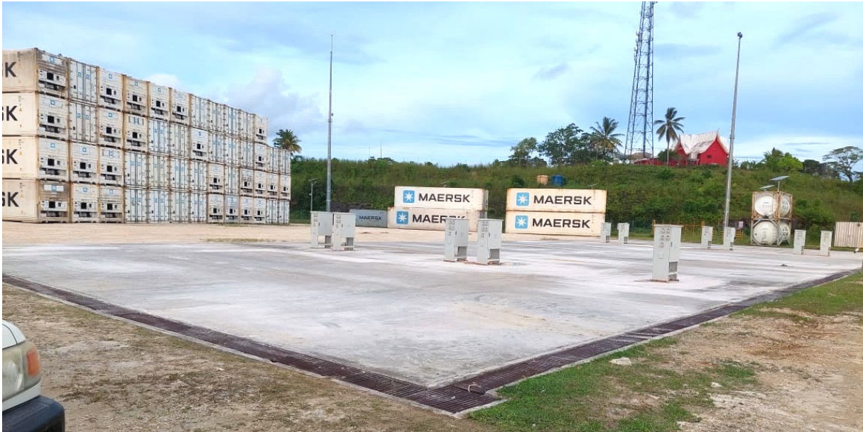
FIGURE 19: PLUG IN AREA AT MAIN PORTS AUTHORITY WHARF, CLOSE ACCESS TO WHARF AND CONTAINER STORAGE YARD
