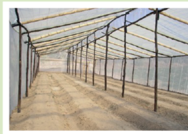
Figure 5. Low-cost greenhouse using a combination of plastic, netting, rough wood and bamboo
