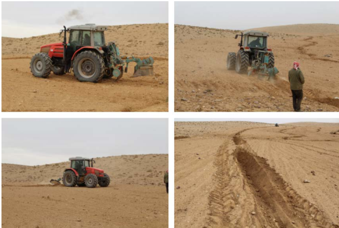
Figure 4.8 | Implementing Vallerani MWH in central Jordan's Badia region
