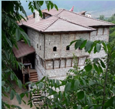
Hupi Tower renovated
