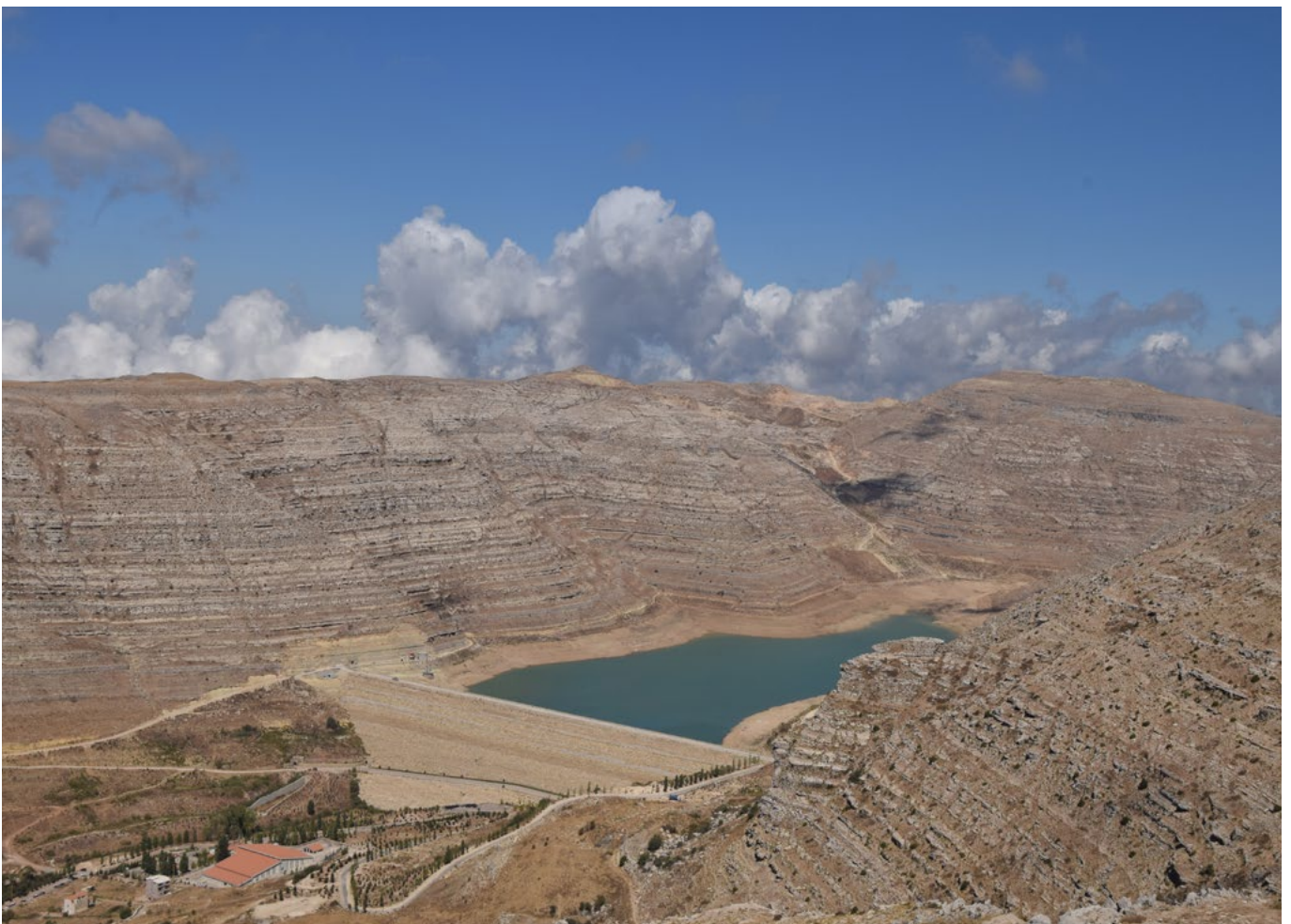
Figure 4. Chabrouh dam, Kalb River Basin, Lebanon
