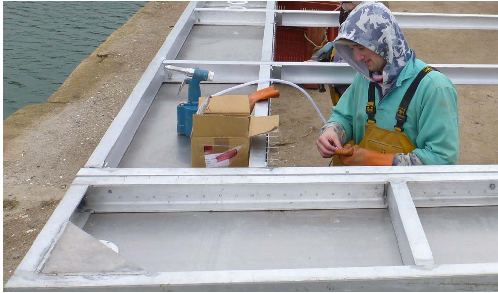
FIGURE 5.20 Riveting the beams onto the side floatation units
