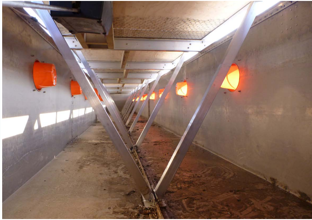
FIGURE 5.26 Diagonal discharge channel supports
