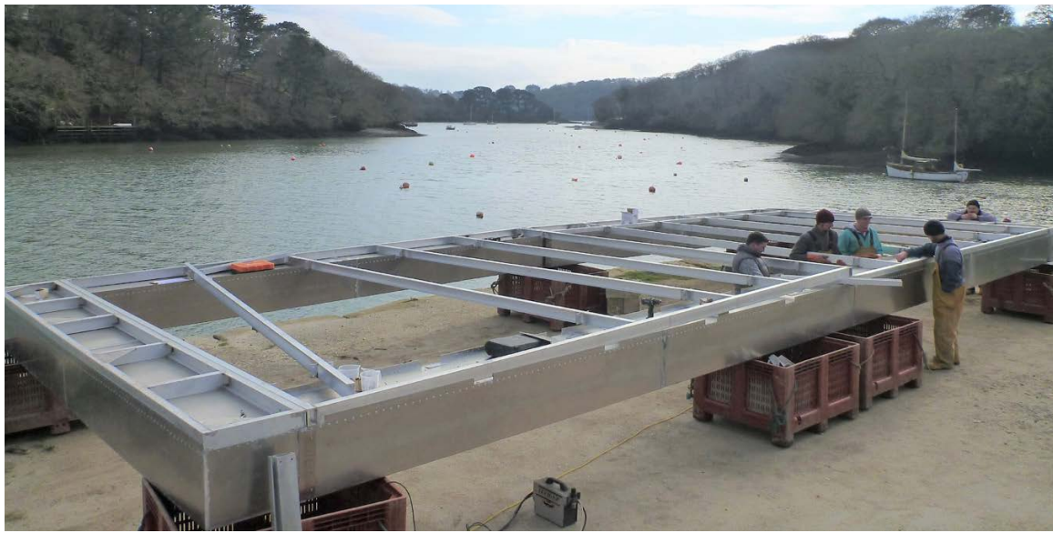
FIGURE 5.16 Laying out the floatation units and loosely bolting together
