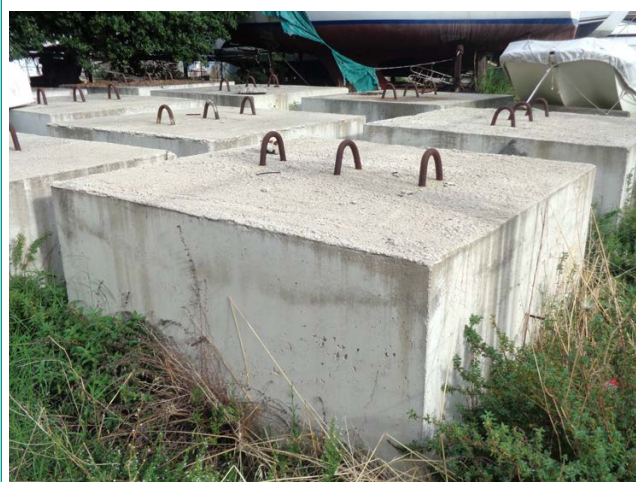
FIGURE 8.5 Long-line mooring concrete blocks
