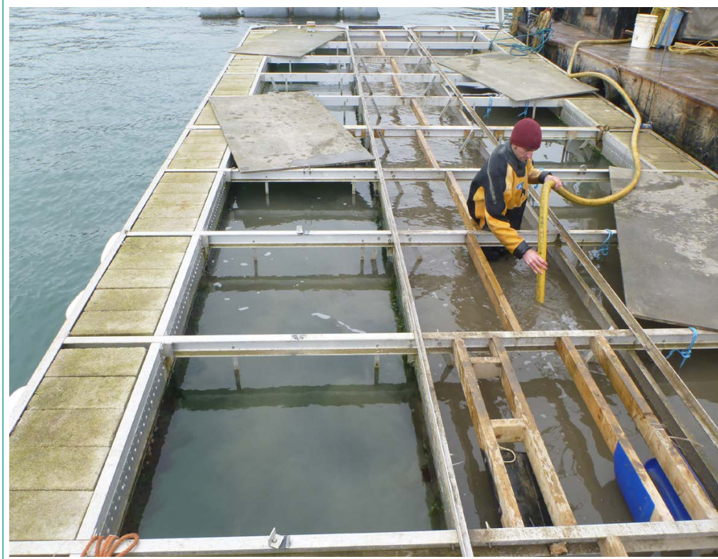
FIGURE 5.5 Central water discharge channel during cleaning process
