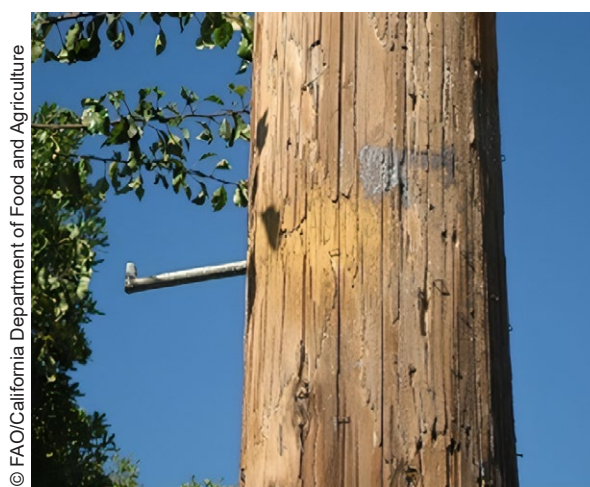
Figure 7.2. Gel application on pole
