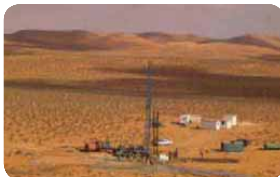
Figure 31: New water point - Tunisia
