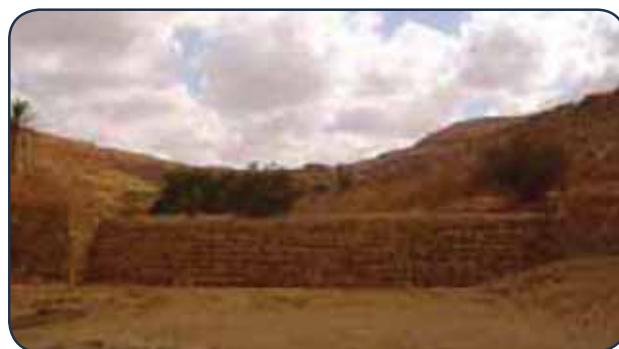
Figure 47: Low cost rehabilitation techniques of water conservation
