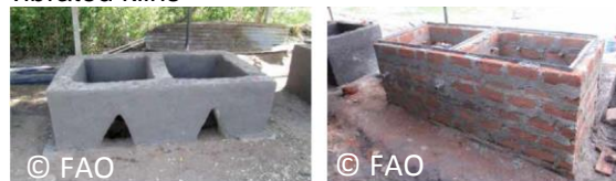
Image 2: Dual compartment frame (left: cement, right: bricks)
