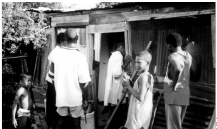
2 Construction of a chicken coop in Bowerbank
