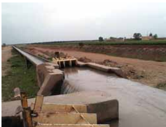
Plate 25 Tail-end spill on a canal equipped with rigid offtakes (baffles), Tadla, Morocco.
