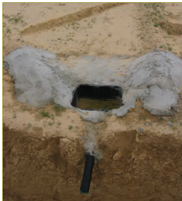
Figure 51: Runoff conveyed to trench through pipe after going through a stilling pond. Mashash Experimental Farm, Israel.
