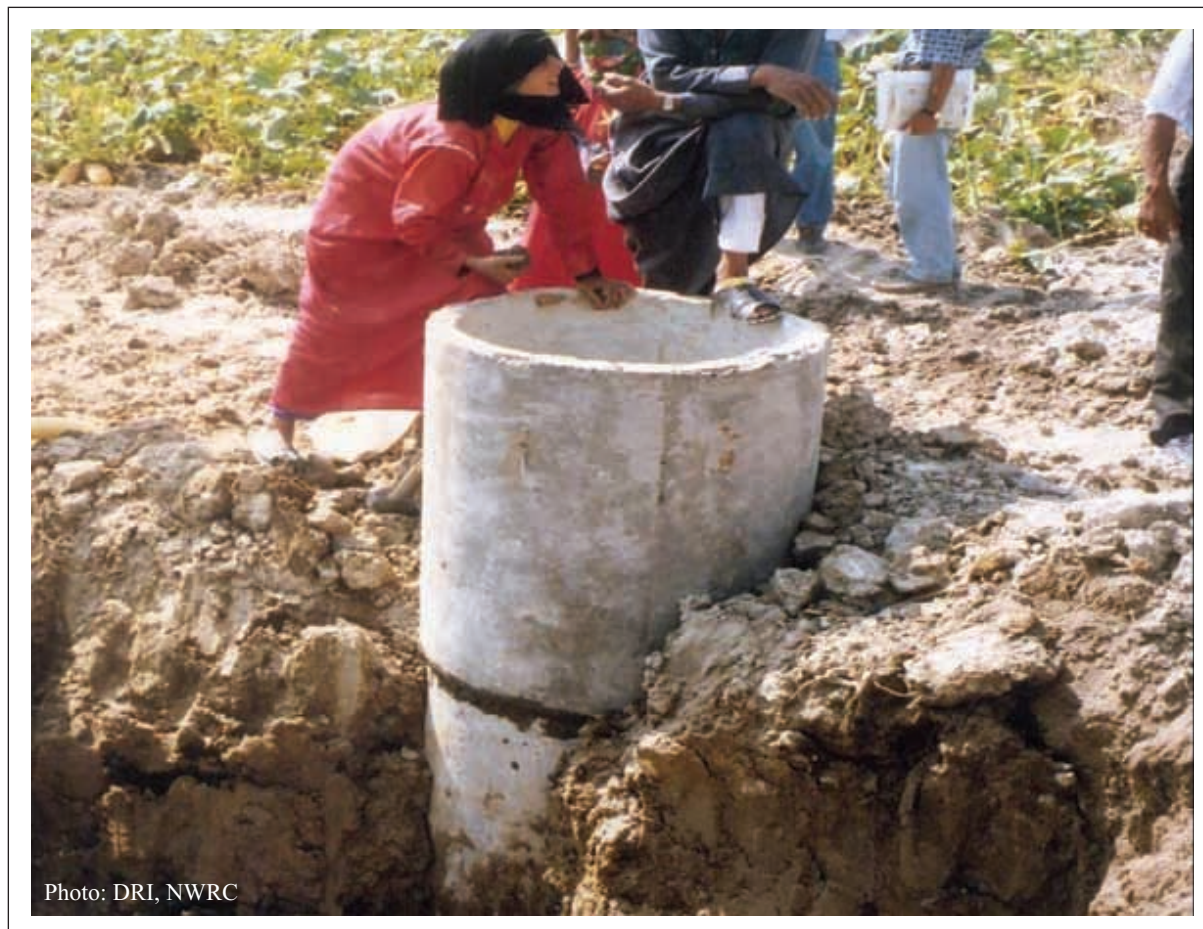
Photo 3: Installation of Pre-Cast Concrete Manholes
