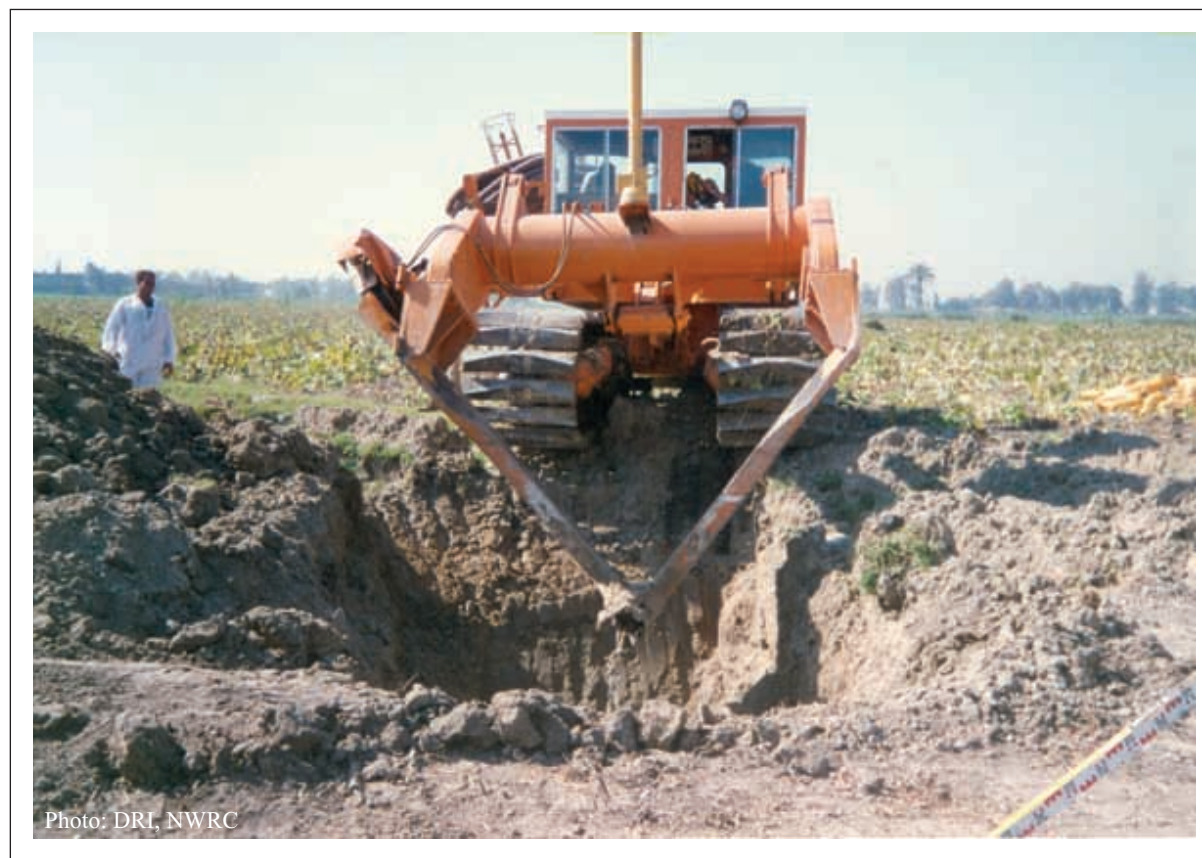
Photo 4: Trenchless Installation Machine
