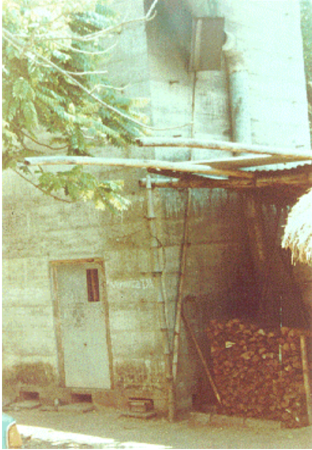
Figure 4. A concrete tobacco curing barn
