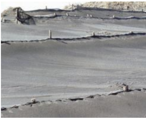
Plate IV Fences erected to catch the drifting sand and rebuild the foredune, preventing the deposition of sand over more inland sites
