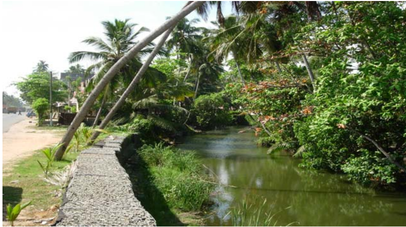
Plate 5.9 Retaining wall to stabilize a roadway: Weligama (Mirissa), Sri Lanka
