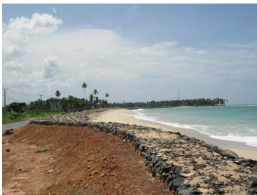
Plate 5.10 Left: Bank revetment, Sri Lanka. Right: Tree planting on the inland side of the revetment
