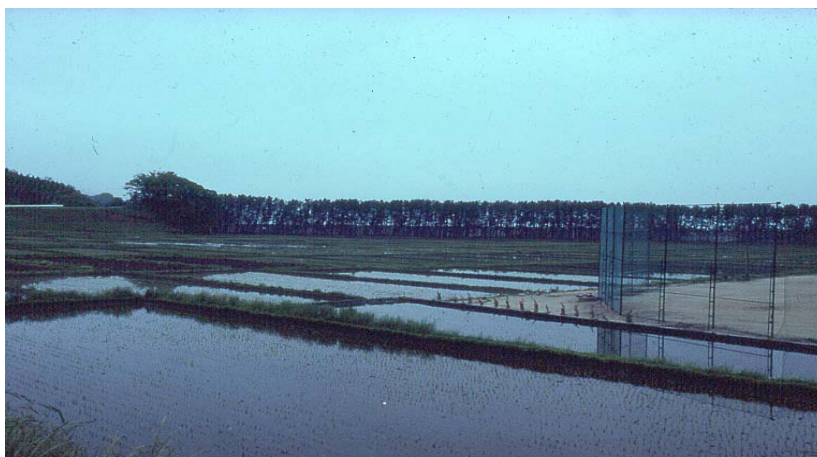
Plate 5.12 Combination of protective planting with agriculture to provide detention for storm water and coastal flooding water (Japan)
