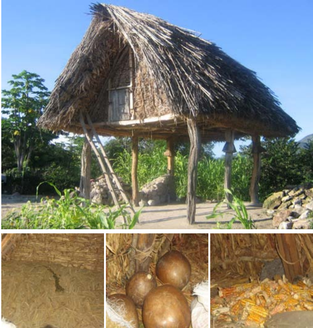
Traditional granary, “Colombier” in French (up) to store and conserve the won crops, particularly harvested grains placed in bulk (down left and right) when not yet picked off, or initially placed in a pre-processed calabash (down center) for better and longer protection. Credits: the Author.
