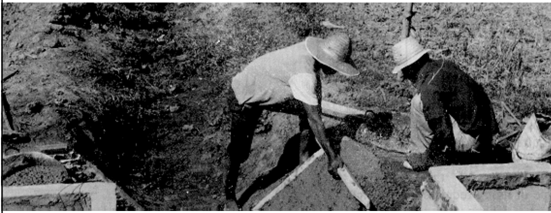
FIGURE 41 Hand plastered canal lining
