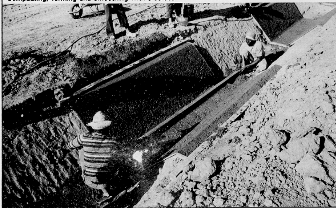
FIGURE 42-C Compacting, forming and smoothing with a screed
