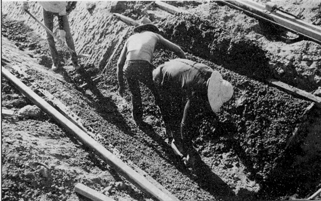
FIGURE 42-B Pouring the concrete
