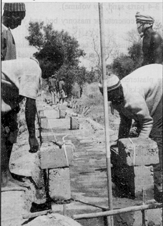
FIGURE 44-C Making the walls
