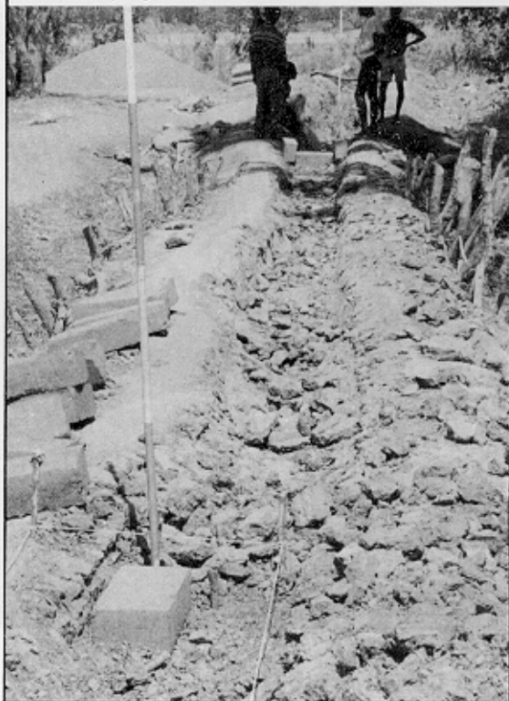
FIGURE 44-A Destroying the old canal bed
