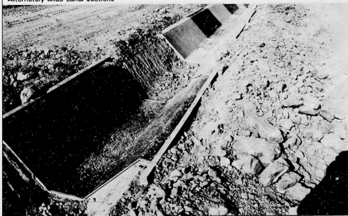
FIGURE 42-D Alternately lined canal sections
