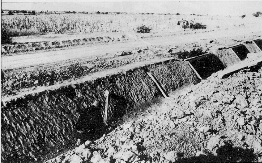
FIGURE 42-A Installation of guide forms
