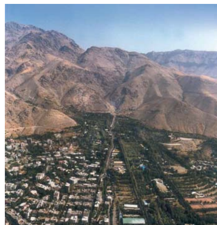
The integration of trees and forests in and around urban areas is an indispensable element of sustainability for the whole society
