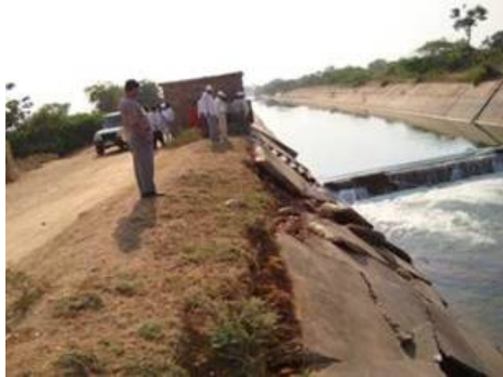
Plate 48. Cross bunding along main canal subsequent to distributaries
