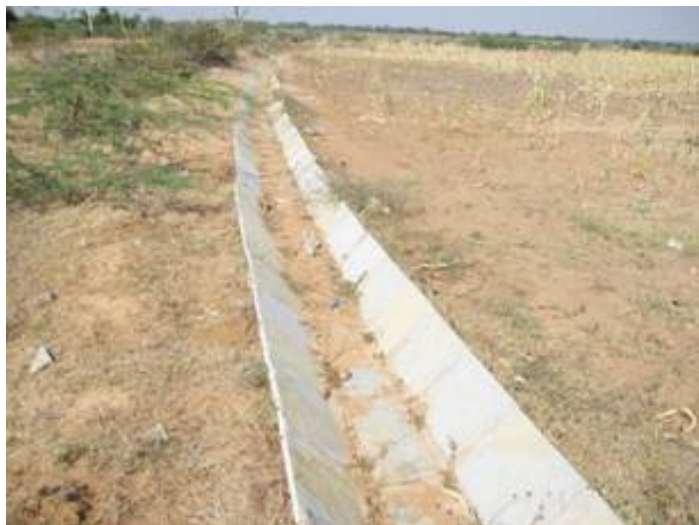
Plate 16 FIC'S without water (left) FIC'S without slab lining (right)
