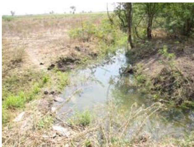
Plate 14 Lateral with damaged lining, weed and jungle growth
