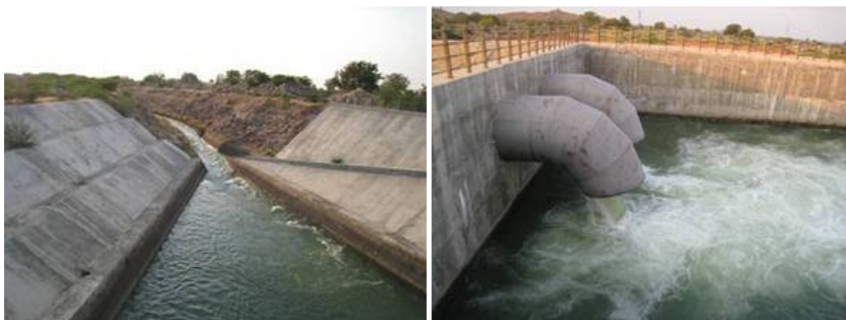
Plate 3. Stage 2 LIFT: Intake of from main canal (left) and Delivery chamber (right).
