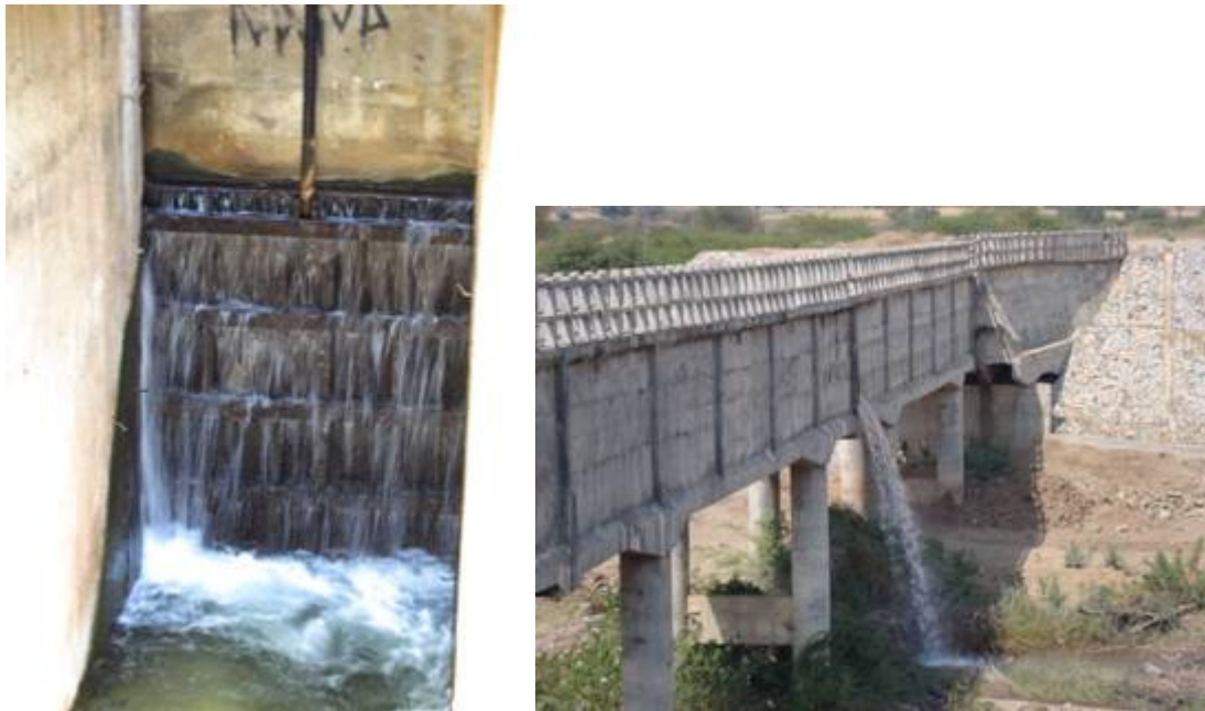
Plate 12. Example of leakages at an escape along SBC (left) on an aqueduct KM 40 OF MBC (right) which are more likely used downstream.
