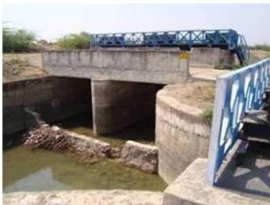
Plate 48. Cross bunding along main canal subsequent to distributaries
