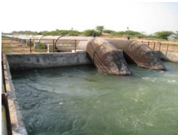
Plate 1. Main pipeline and delivery chamber of one lift system in Rampur
