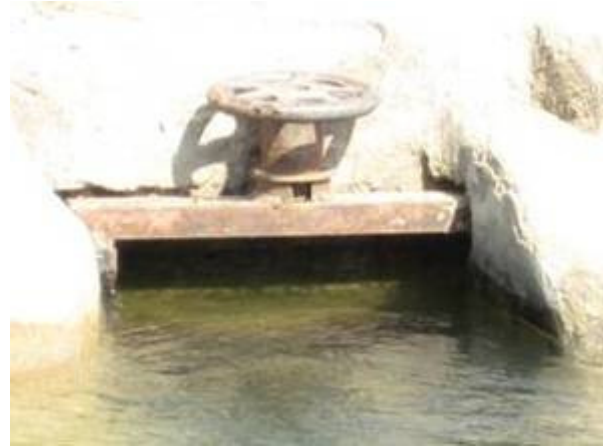
Plate 19 Damaged gate for D.P.O
