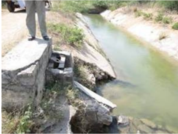
Plate 18 Damaged gate for lateral
