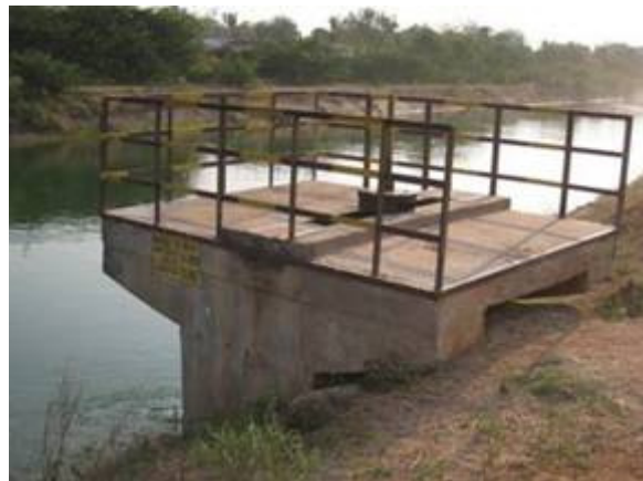
Plate 41 Cross regulator and main offtake along NRBC
