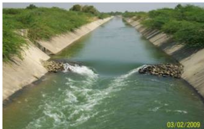
Plate 6. Lack of water level control compensated by temporary weirs made of rocks
