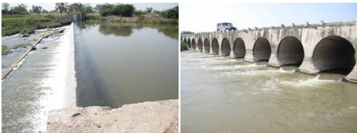
Plate 11 Downstream of Shahapur BC, weir with possibility of monitoring the flow (left) – bridge which should be equipped with measurement device (right)
