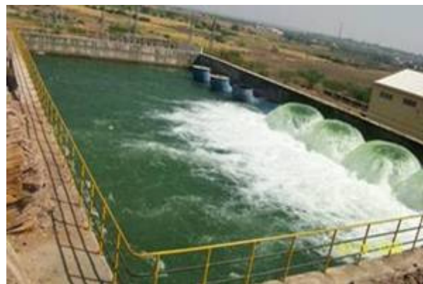
Plate 5. Raising pipes and delivery chambers at ILIS
