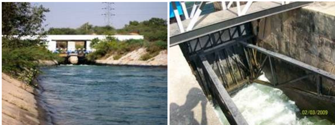
Plate 9. D/S of the SBC Head Regulator View showing the Radial gate
