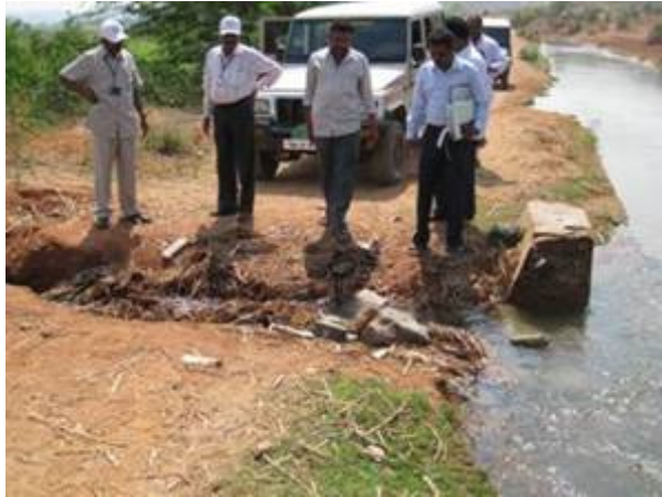
Plate 40 Ungated distribution along secondary and laterals
