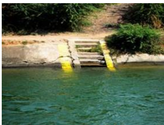
Plate 20 Gauge painted on SBC
