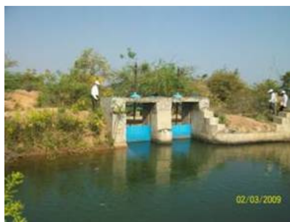
Plate 24 Cross Regulator Cum Escape Km 13.70 of SBC Plate 25 Cross Regulator Cum Escape Km.- 7.5 of Dy.-6
