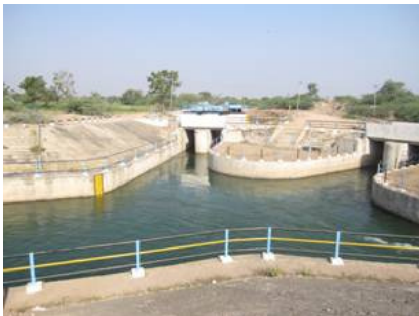
Plate 10 Y- Junction structure comprising MBC, SBC and Escape.
