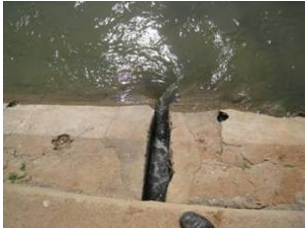
Plate 40 Ungated distribution along secondary and laterals
