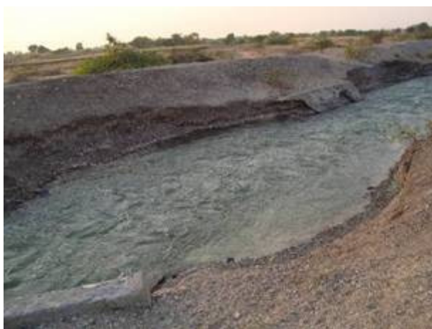
Plate 45. Scouring of canal lining in JBC DY-12
