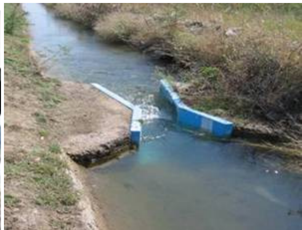
Plate 57 Measurements flumes
