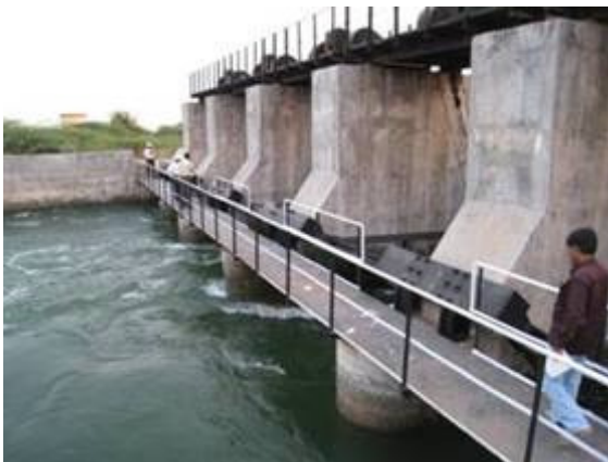
Plate 41 Cross regulator and main offtake along NRBC
